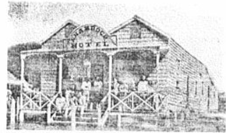
39 Shamrock, formerly European (Flinders Street), c. 1875. Typical of single-storyed hotels not on a corner in having twin gables facing the street. It was typical in having a verandah behind the street alignment.
